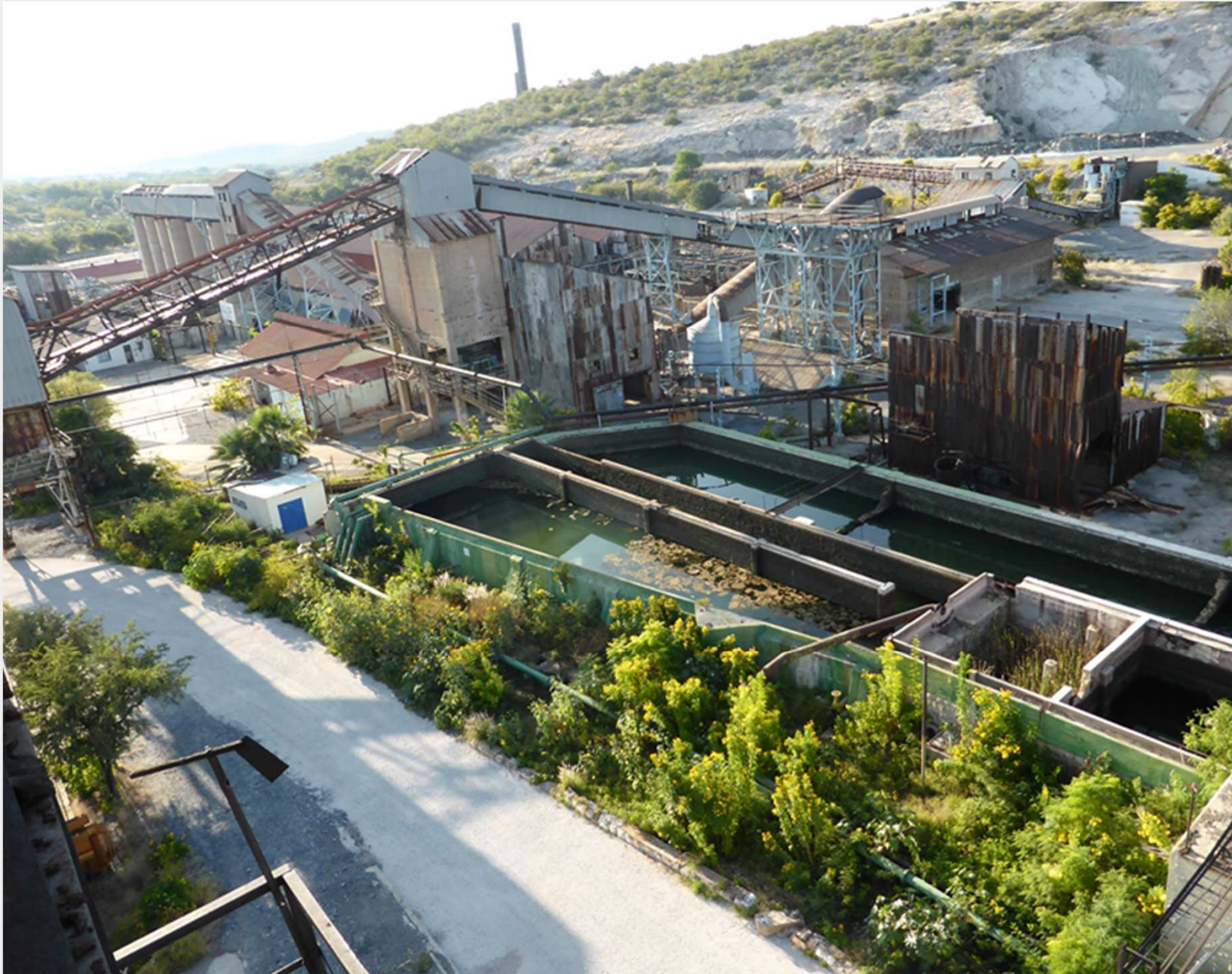
VIEW FROM PLATFORM: DISTRICT OF FORMER BENEFICIATION OF THE ORE; OPEN PIT IN BACKGROUND
